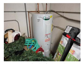
This is an A.O. Smith, 60 gallon electric water heater (installed October 2013).
