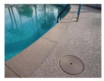
The acrylic pool deck was resurfaced in January 2018. This component budgets to repair & recoat (repaint) the pool deck on a six (6) year cycle.
