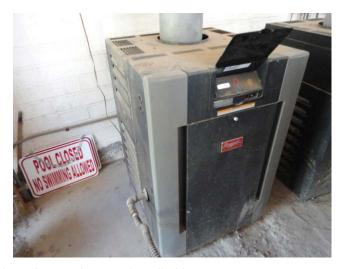
This is a Raypak, 400,000 BTU input heater that was installed in 2013.
