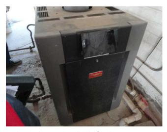
This is a Raypak, 400,000 BTU input heater that was installed in October 2016.
