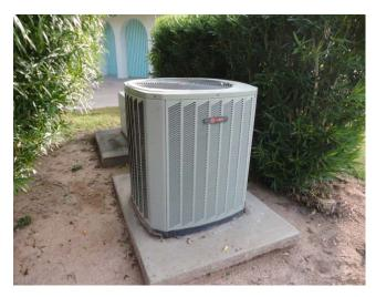
This is a Trane, 5 ton split system that was installed in August 2011 at a cost of \$6,887.68.
